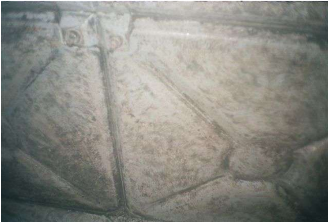
These pictures show the internal substrate of tank #2 after being prepared by COVAC Operatives.
