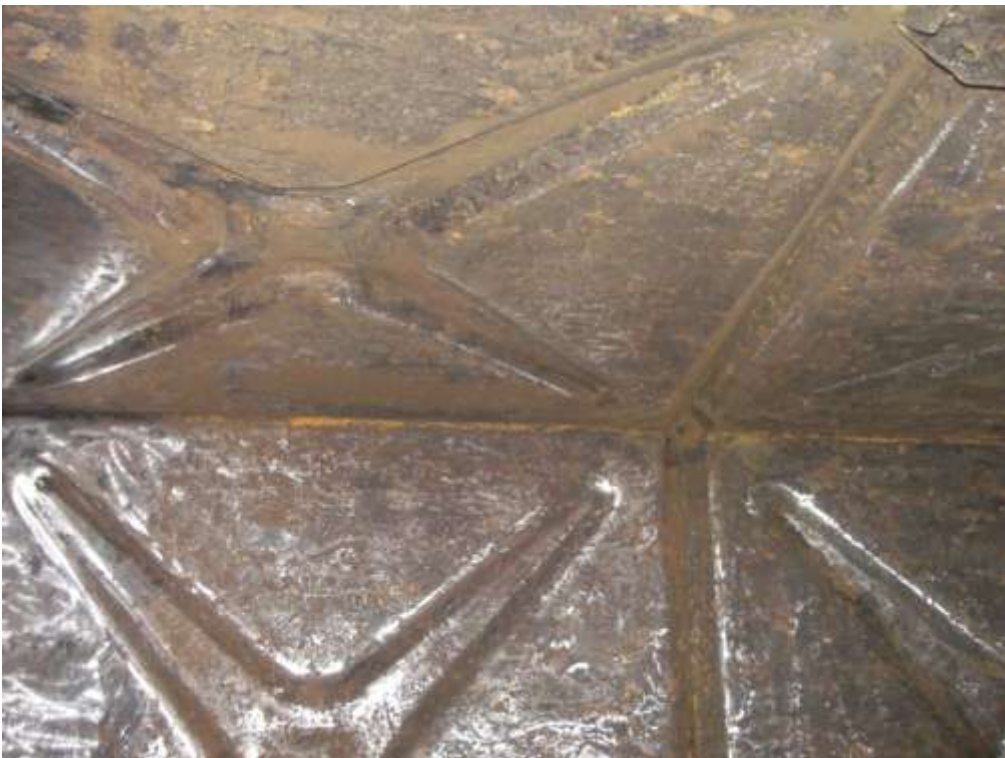
These pictures show the internal substrate of tank #1 after being prepared by COVAC Operatives.
