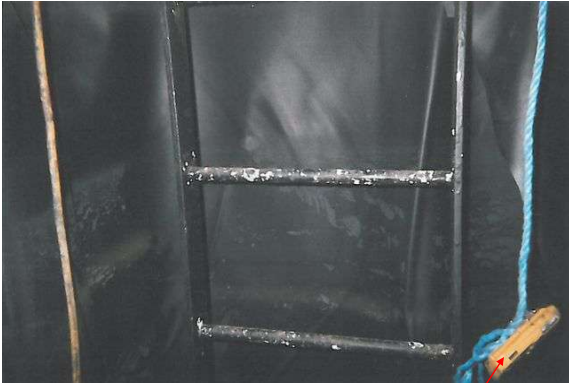
Gas Alert Monitor
