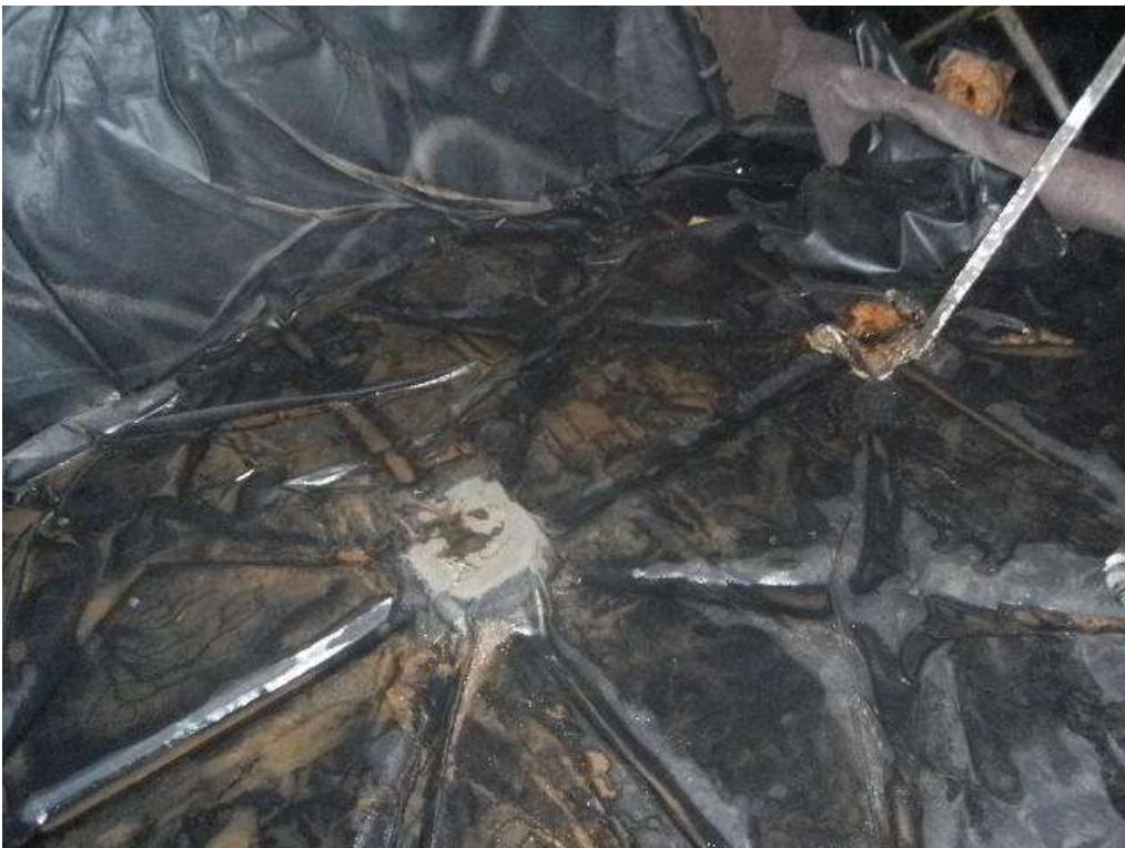
These images show the tank after being drained of water and before / during removal of the failed butyl liner, felt lining and insulation.
