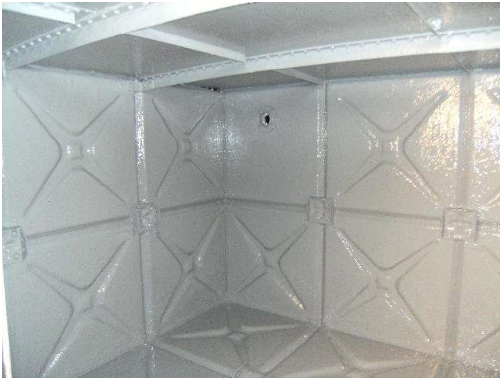
The following photographs show the final application of the 2 nd coat of 3M Scotchkote™ 165PW (grey).
