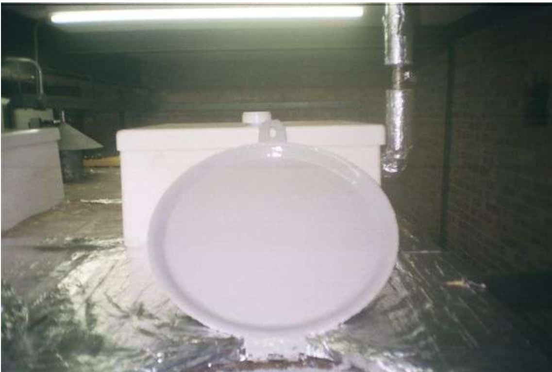
The existing hatch covers were also coated.
