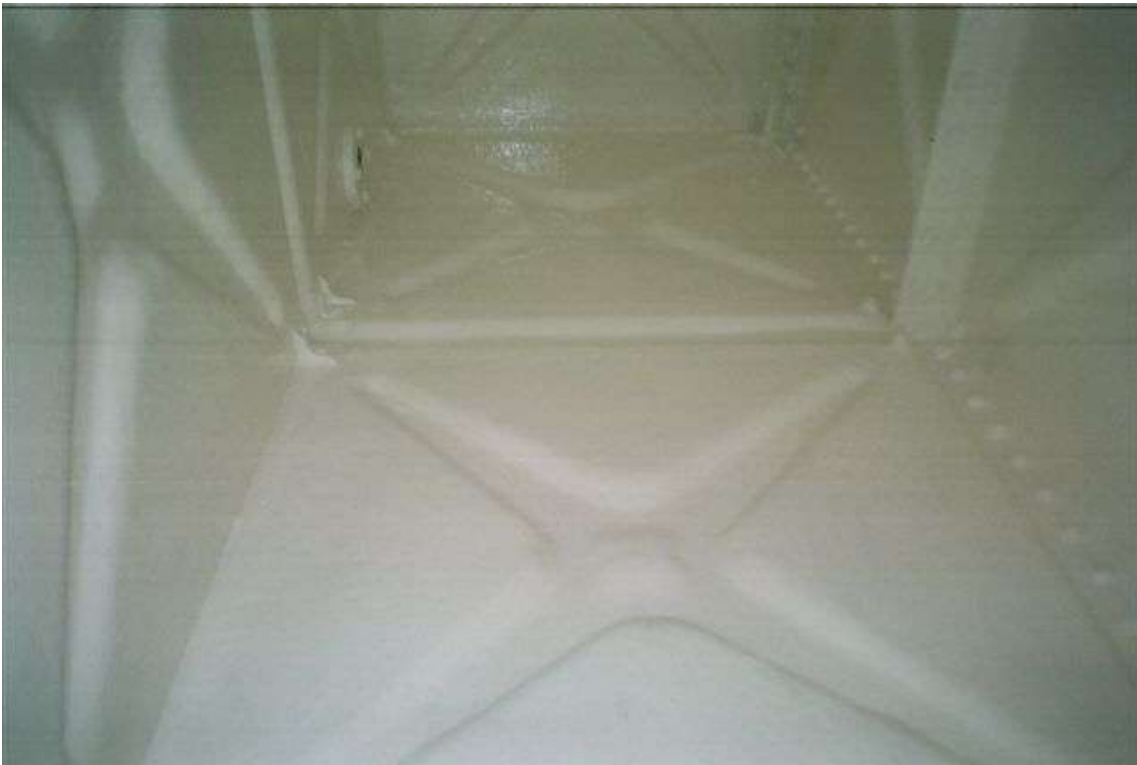
All seams, joints, bolts etc were initially 'stripe coated' to ensure all intricate areas were coated. These photographs show the substrates having received the 1 st full coat of 3M Scotchkote™ 165PW (cream).
