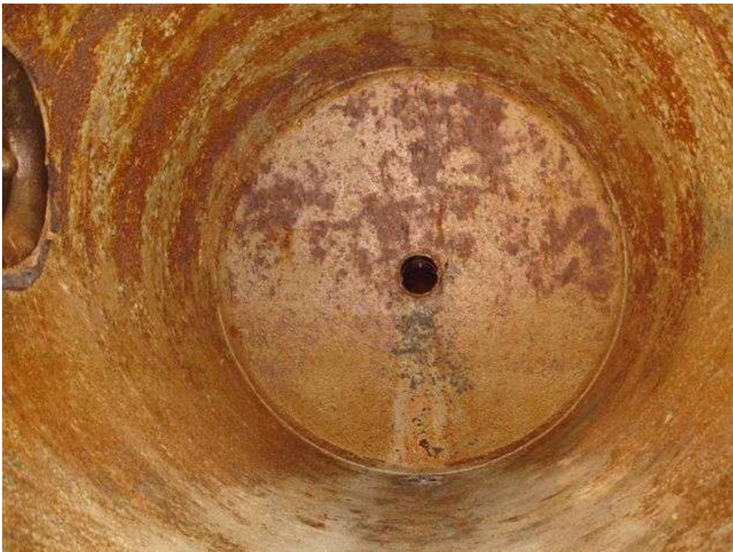
These photographs show the internal surfaces of the vessels having been drained of water and prior to any preparation works being carried out.
