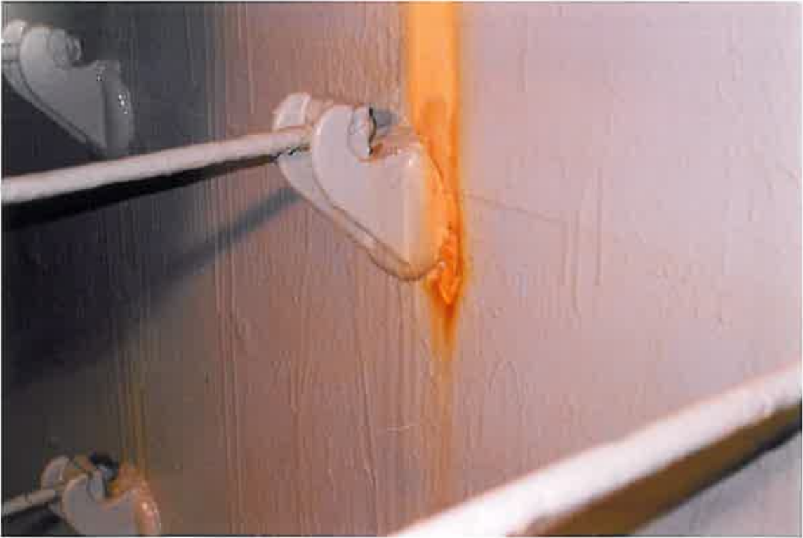
These photographs show the tanks internals drained of water and prior to any preparation.
