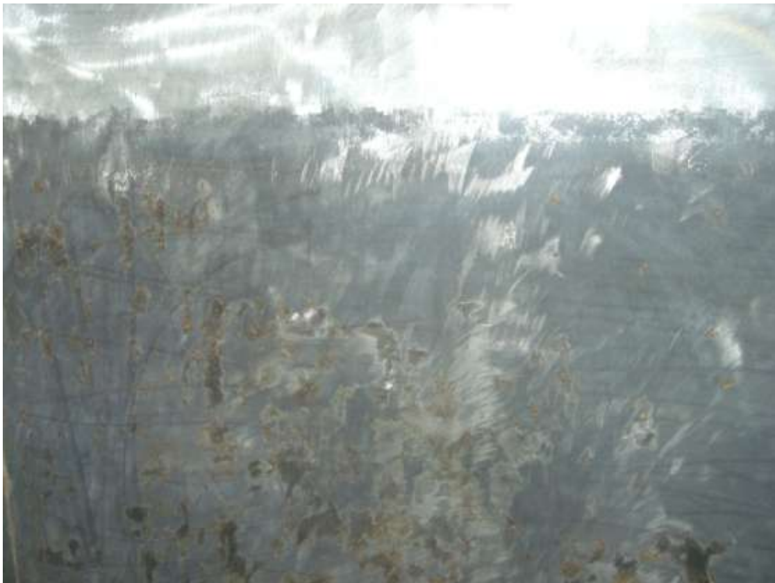
The pictures show the internal substrate after being prepared by COVAC Operatives.
