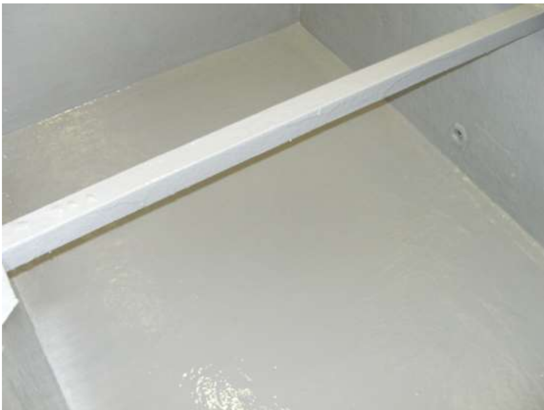
The following photographs show the final application of the 2 nd coat of 3M Scotchkote™ 165PW (grey) in order to achieve a total, nominal dry film thickness of 1000 Microns (1mm), and between 1500-2000 Microns (2mm) over all stripe coated areas.
