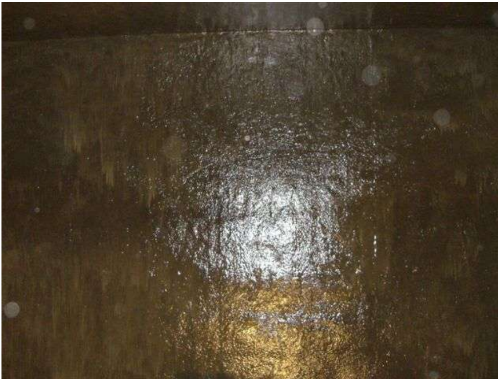
These photographs show the application of 3M Scotchkote™ 165PW Clear Sealer.
