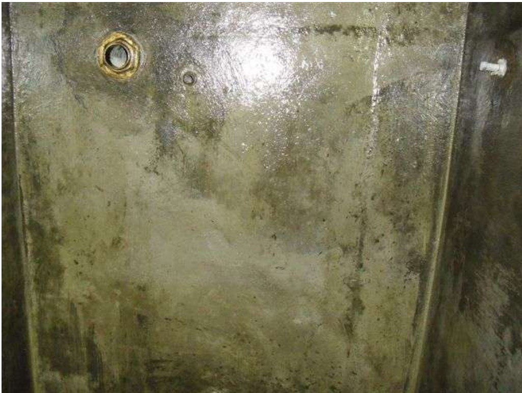
These pictures show the structure after the application of 3M Scotchkote 165PW Clear Sealer to all surfaces.
