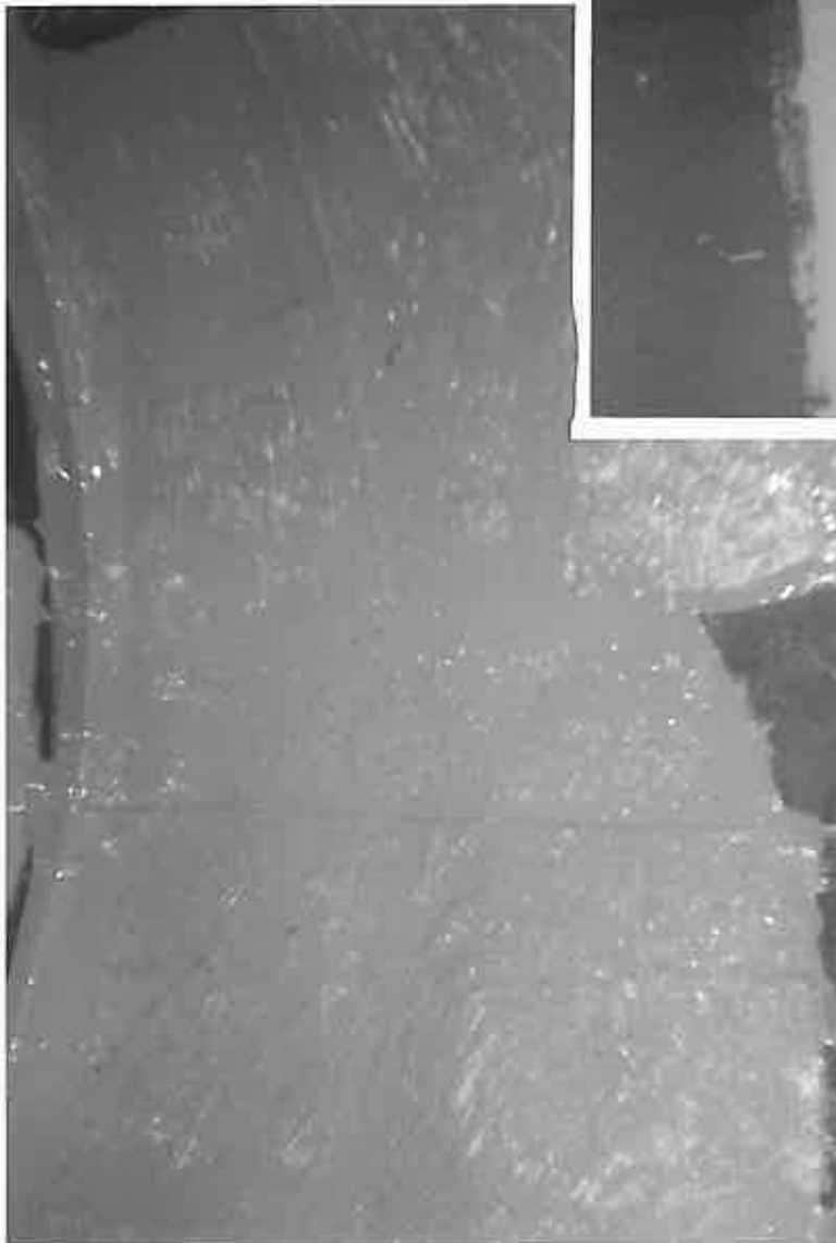
These photographs show fibreglass reinforced bandaging was used in conjunction with a full coating of COPON Hycote 165PW Solvent Free Polyurethane (cream) over severely corroded areas.
