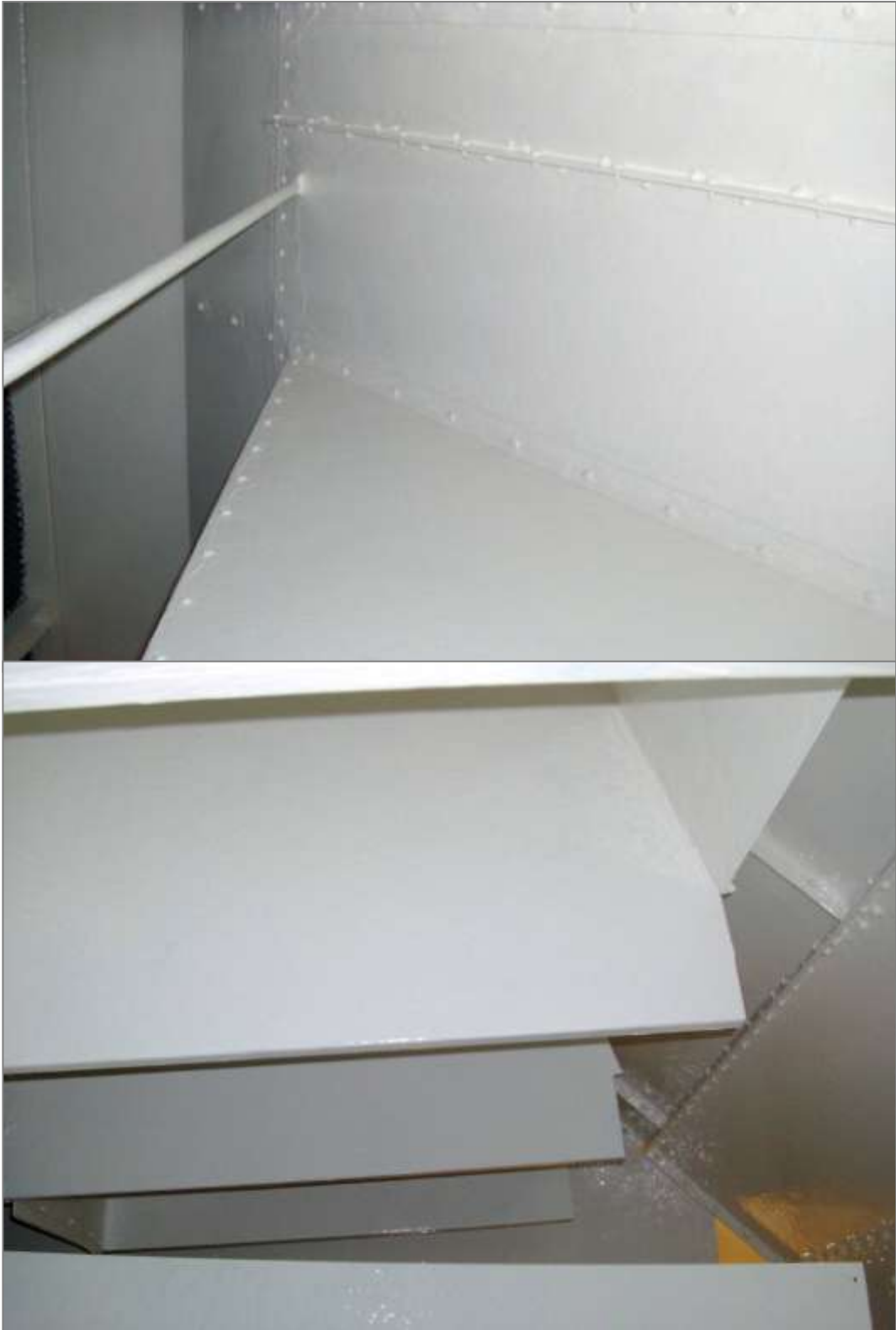
These photographs show the substrate having received the 1 st coat of 3M Scotchkote™ 165PW (cream) Solvent Free Polyurethane.
