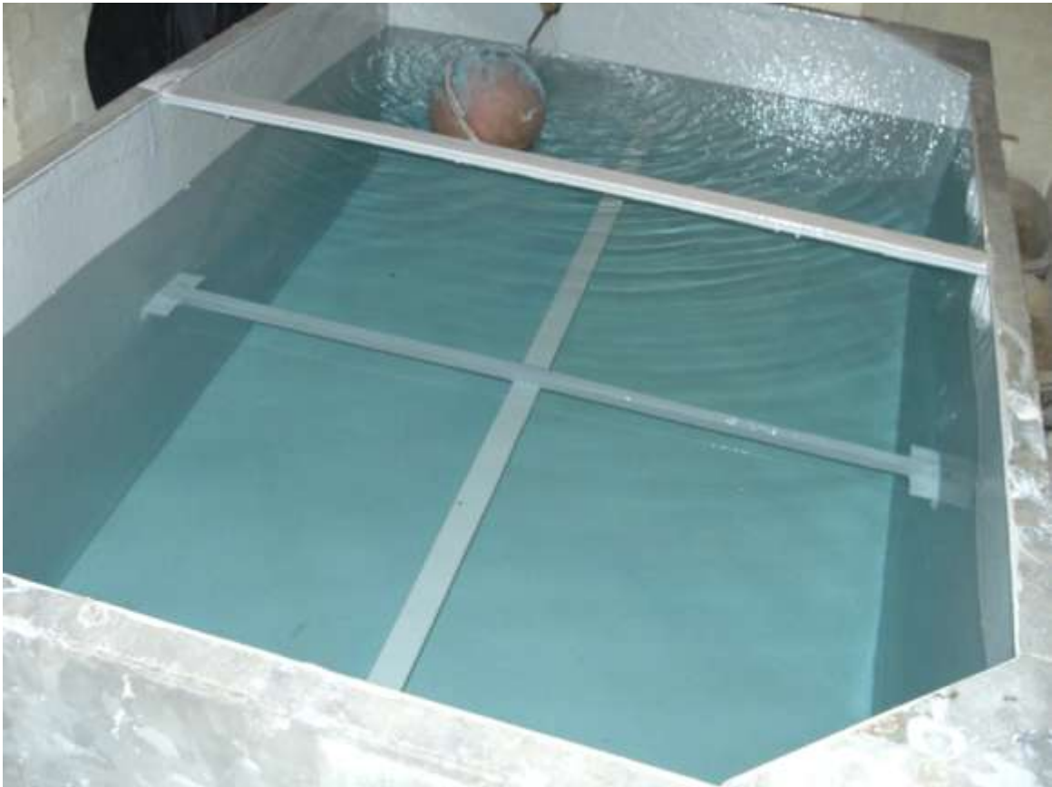
These images show the completed tanks refilled with water.
