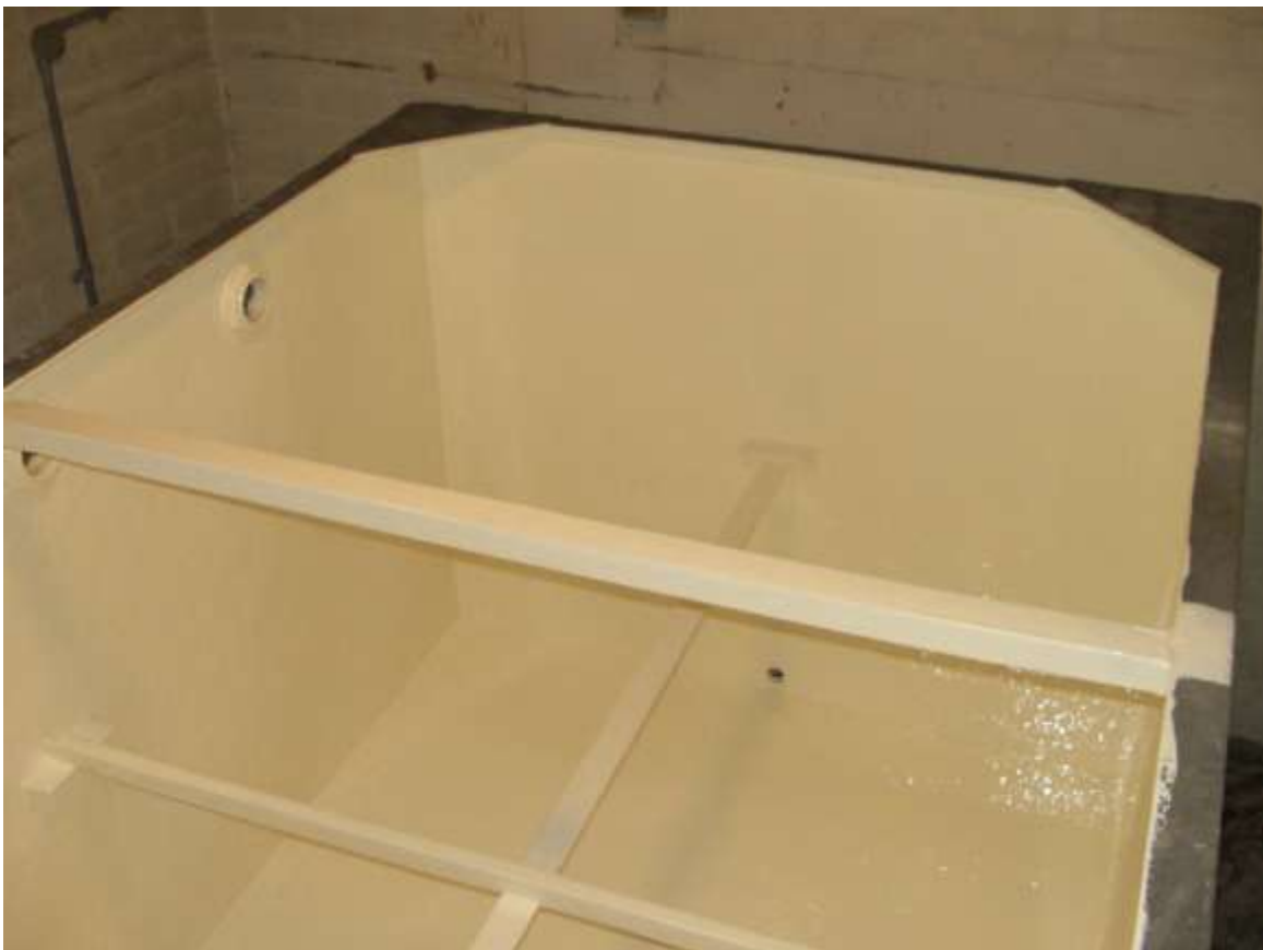
These photographs show the substrate of the tanks having received the 1 st full coat of 3M Scotchkote™ 165PW (cream) Solvent Free Polyurethane, by means of brush and roller to a nominal wet/dry film thickness of 500 Microns.
