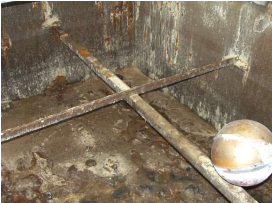
These photographs show the internal surfaces of the tanks having been drained of water and prior to any preparation works being carried out. The corrosion within the tanks is clearly evident.
