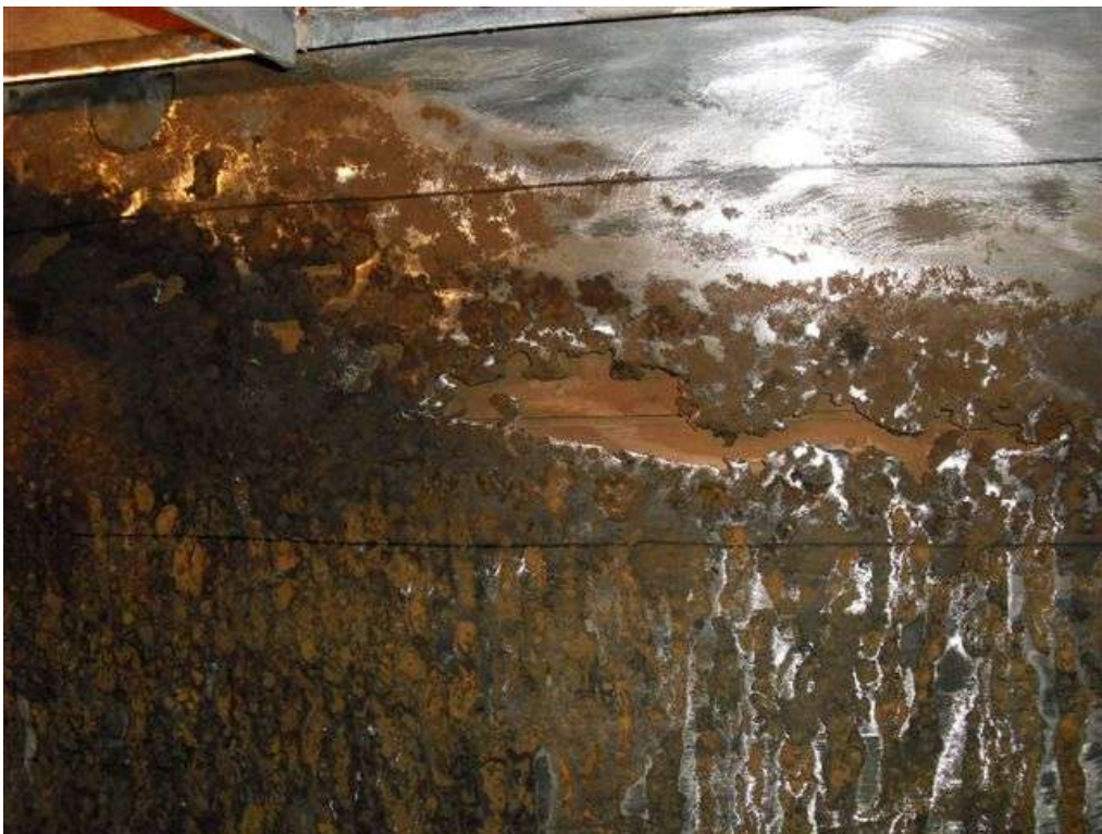
These pictures show the internal substrate after being prepared by COVAC Operatives, in accordance with ISO 8501-1:2007, utilizing mechanical power tools and manual tools. The holes can be more clearly seen after preparation and were marked out before 'stripe coating' utilising 3M Scotchkote™ 165PW.
