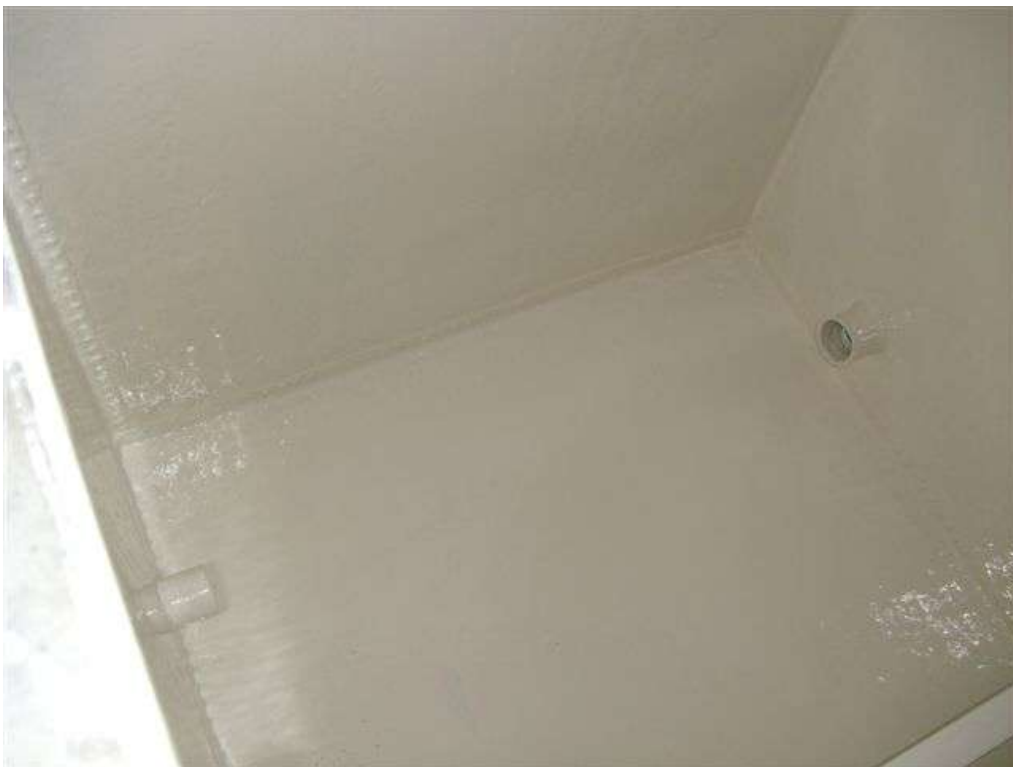
These photographs show the substrates having received the 1 st full coat of 3M Scotchkote™ 165PW (cream) Solvent Free Polyurethane, by means of brush and roller to a nominal wet / dry film thickness of 500 Microns.
