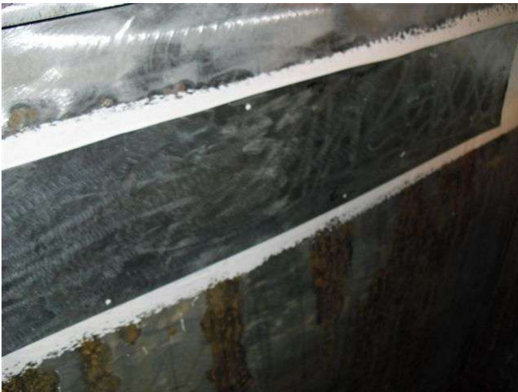
Steel plates were then fastened to the damaged areas.
