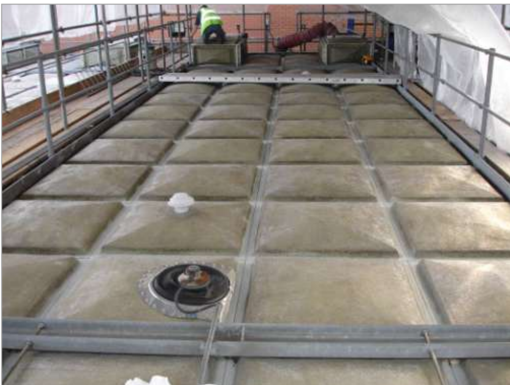
These pictures show the external roof joints of the structure being prepared by COVAC Operatives in order to raise a suitable surface profile to promote optimum adherence of the 3M Scotchkote™ 165PW system.
