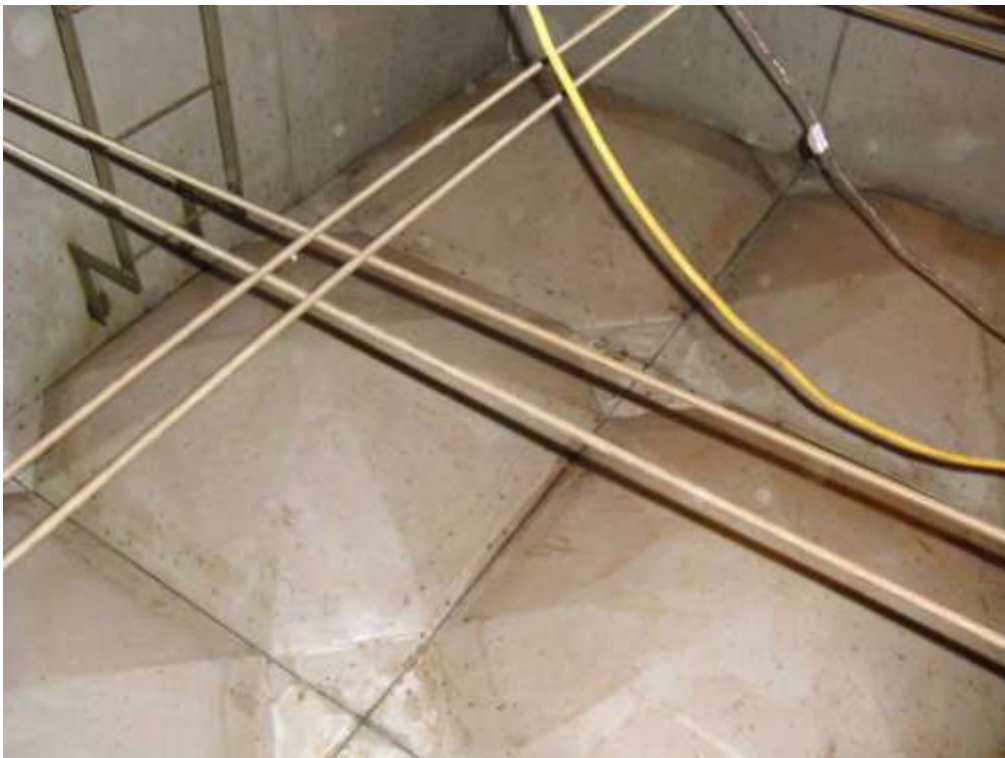
These photographs show the internal surfaces of the tank having been drained of water and prior to relining work commencing. Black spore fungi can be clearly seen over much of the substrate.
