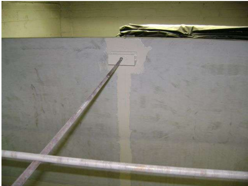
All joints were treated to prevent leaks and allowed to cure.
