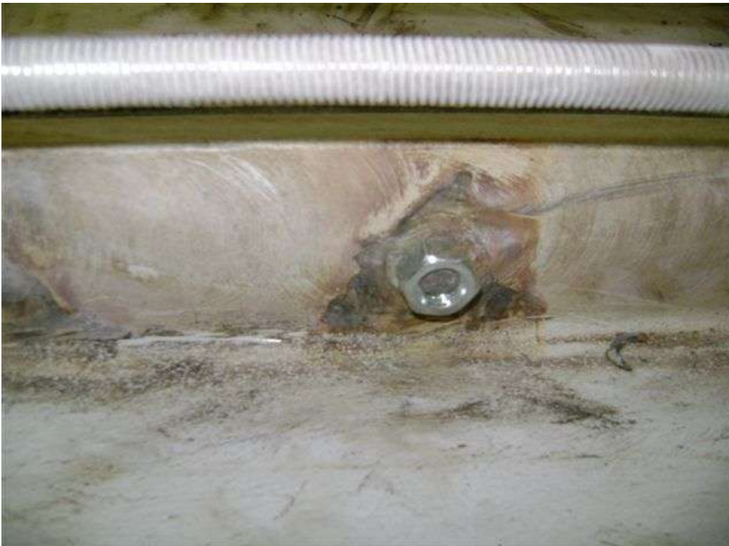
These pictures show the internal substrate after being prepared by COVAC Operatives in order to raise a suitable surface profile on the substrate and promote optimum adherence of the 3M Scotchkote™ 165PW lining system.
