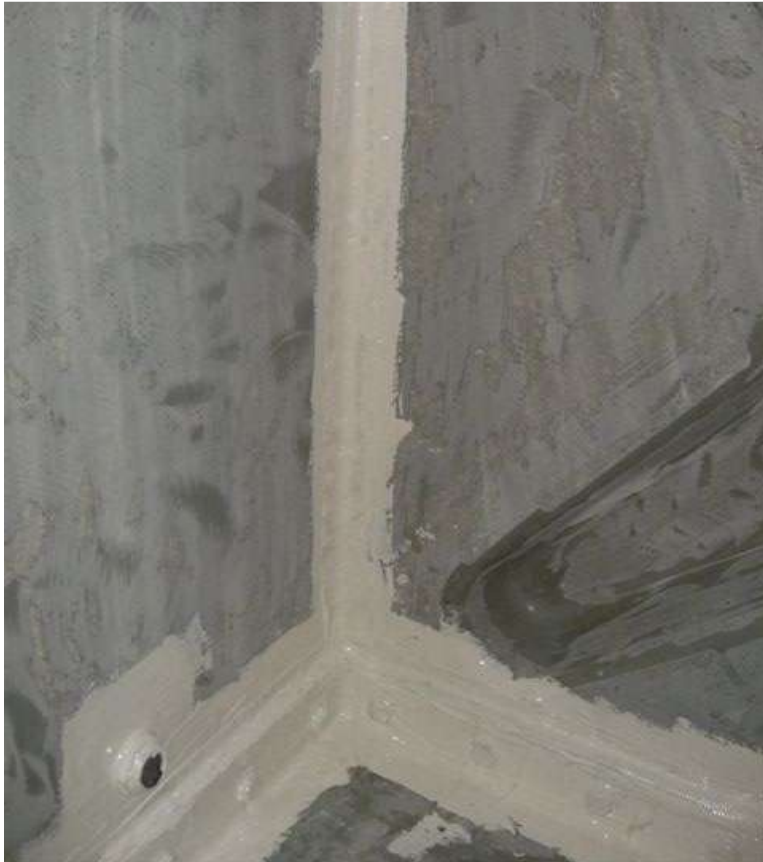
All joints were treated to prevent leaks and allowed to cure.
