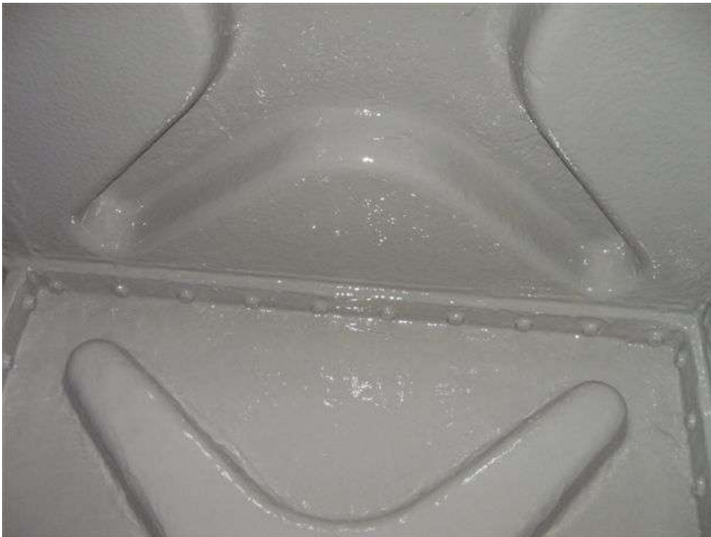
The following photographs show the final application of 3M Scotchkote™ 165PW (grey).
