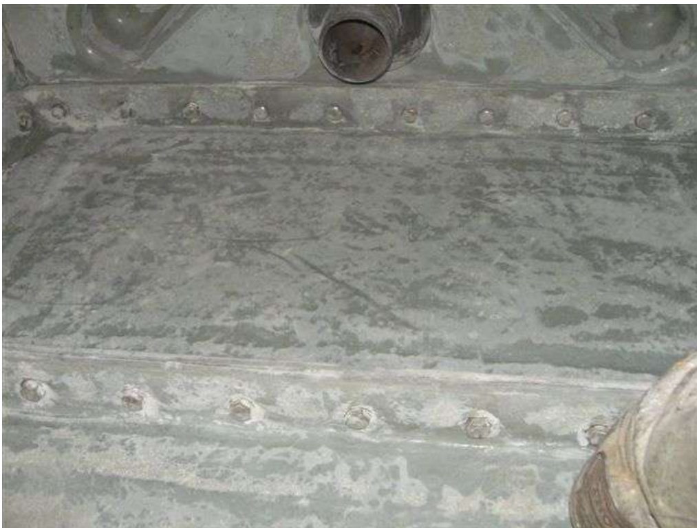
These pictures show the internal substrate of the tank after preparation by COVAC Operatives, in order to raise a suitable surface profile on the substrate and promote optimum adherence of the 3M Scotchkote™ 165PW lining system.
