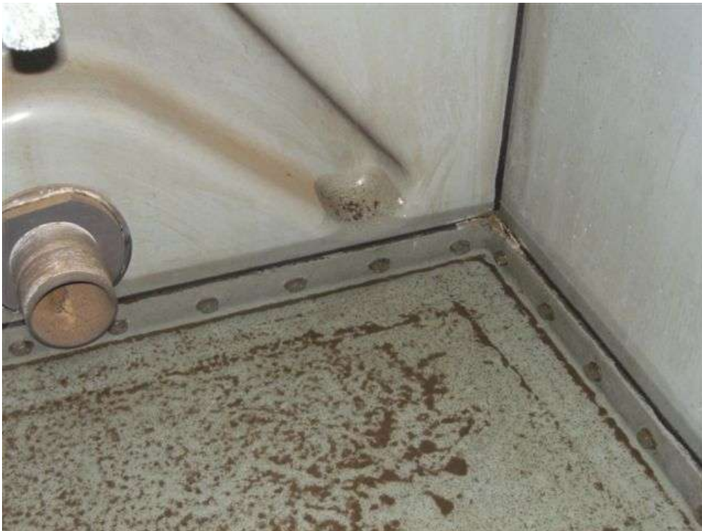
These photographs show the internal surfaces of the tank having been drained of water, but prior to any work commencing.
