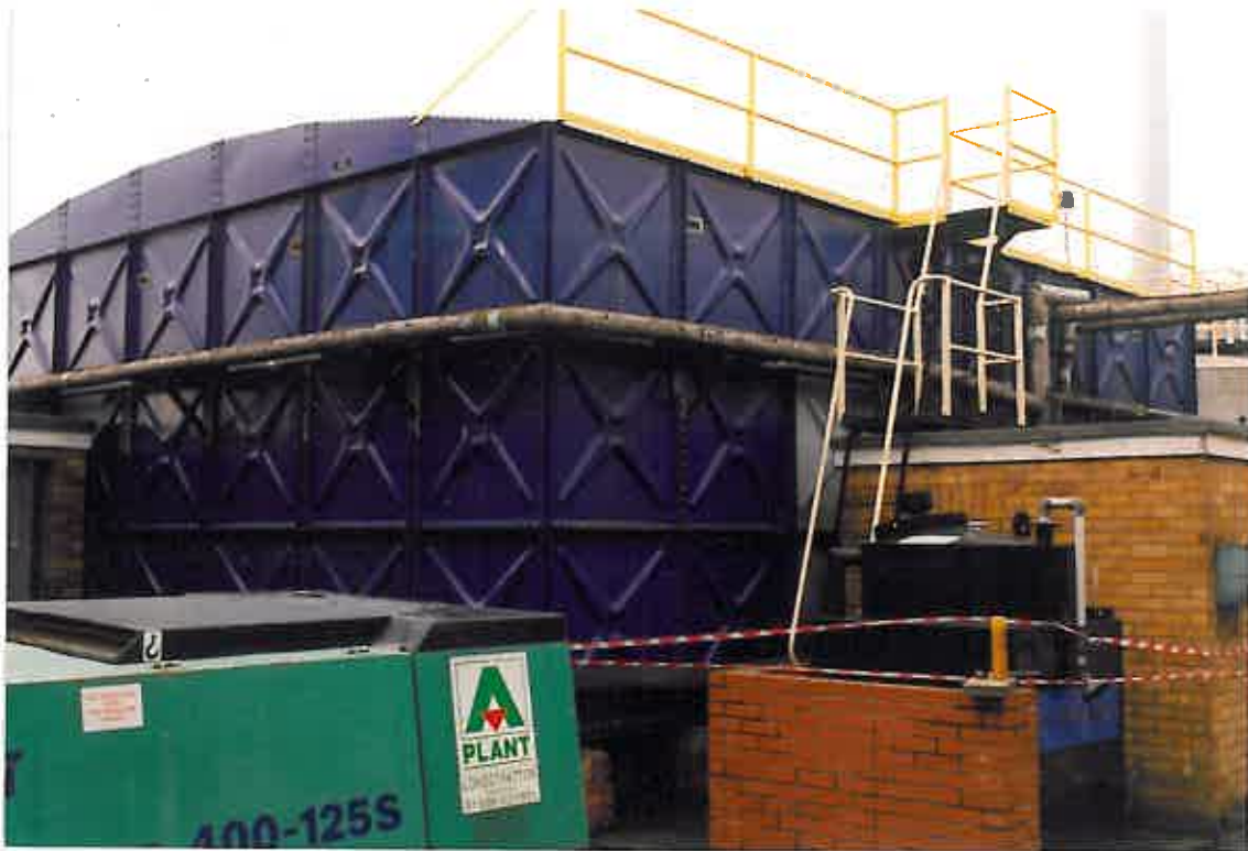
These photographs show the external of the tank
