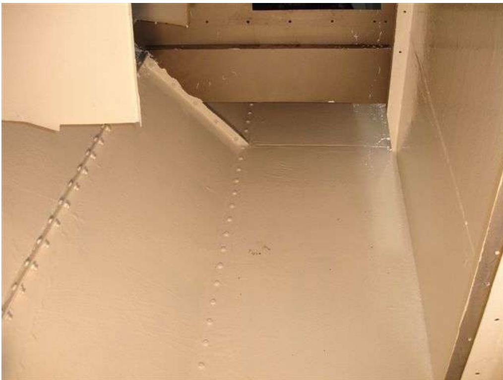
These photographs show the substrates having received the 1 st full coat of 3M Scotchkote™ 165PW (cream) Solvent Free Polyurethane.
